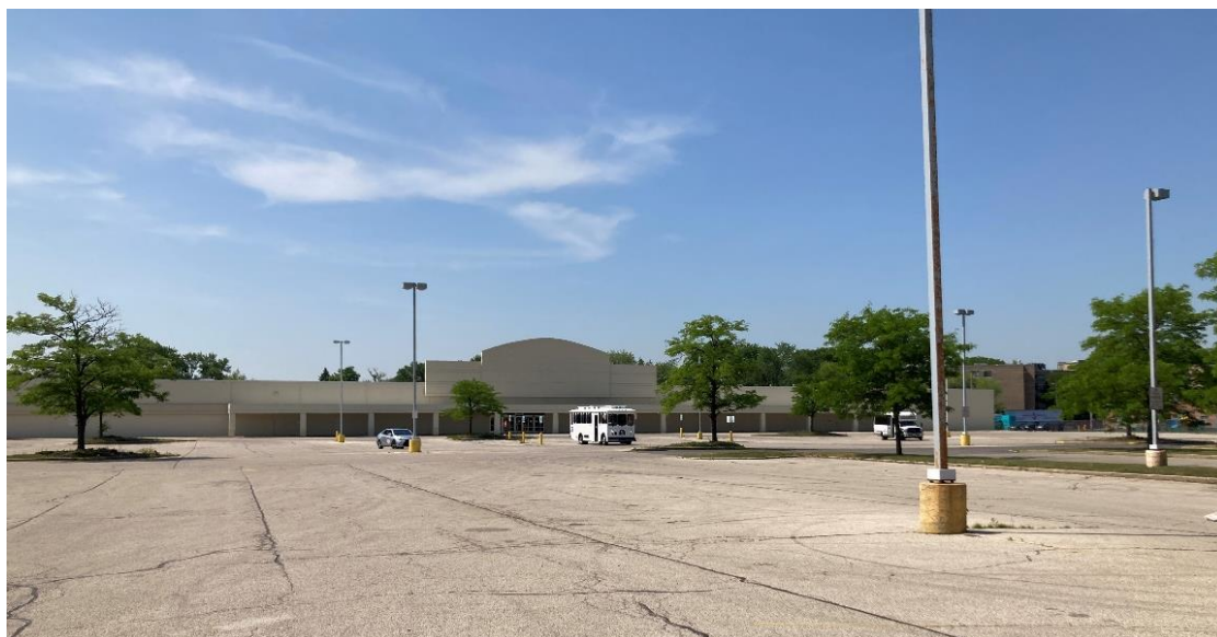
View of the Kmart site, looking south. June 2, 2023.
